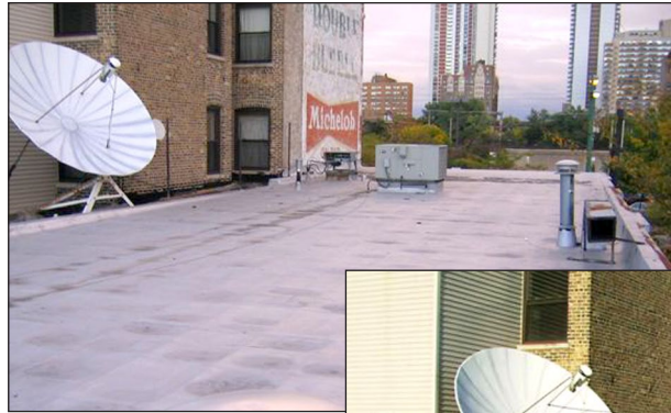
Roof of an organic grocery store in Chicago before and after planting
