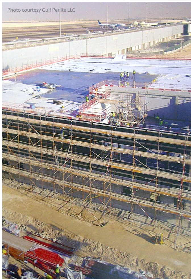
Figure 1 • Abu Dhabi Airport Terminal roofing with perlite lightweight insulating concrete stand-alone insulation.
