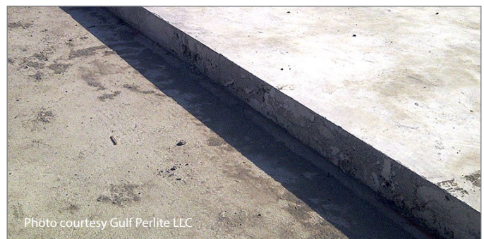
Top: Placing and screeding a perlite lightweight concrete roof deck. Above: Strong, smooth, monolithic surface of a perlite lightweight concrete roof deck installation.
