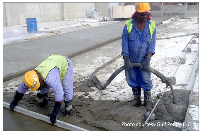
Figure 2 (left) • Cross-section of 3-hour fire-rated roof deck with application of perlite lightweight concrete.
