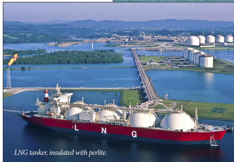
LNG storage tanks insulated with perlite.
