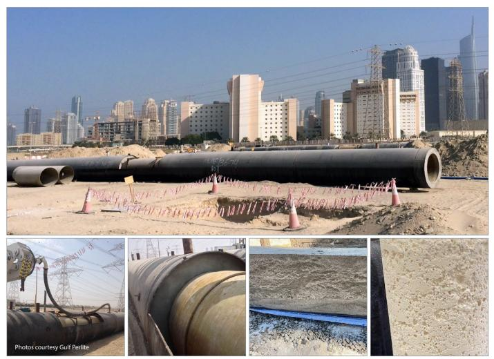
Perlite concrete pipe insulation provides a seamless, lightweight, quality thermal insulation that is also fire, rot, and vermin proof.
