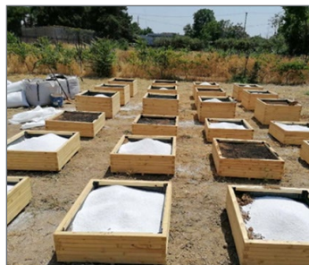
Figure 5 • Construction phase: fine perlite addition in containers.
